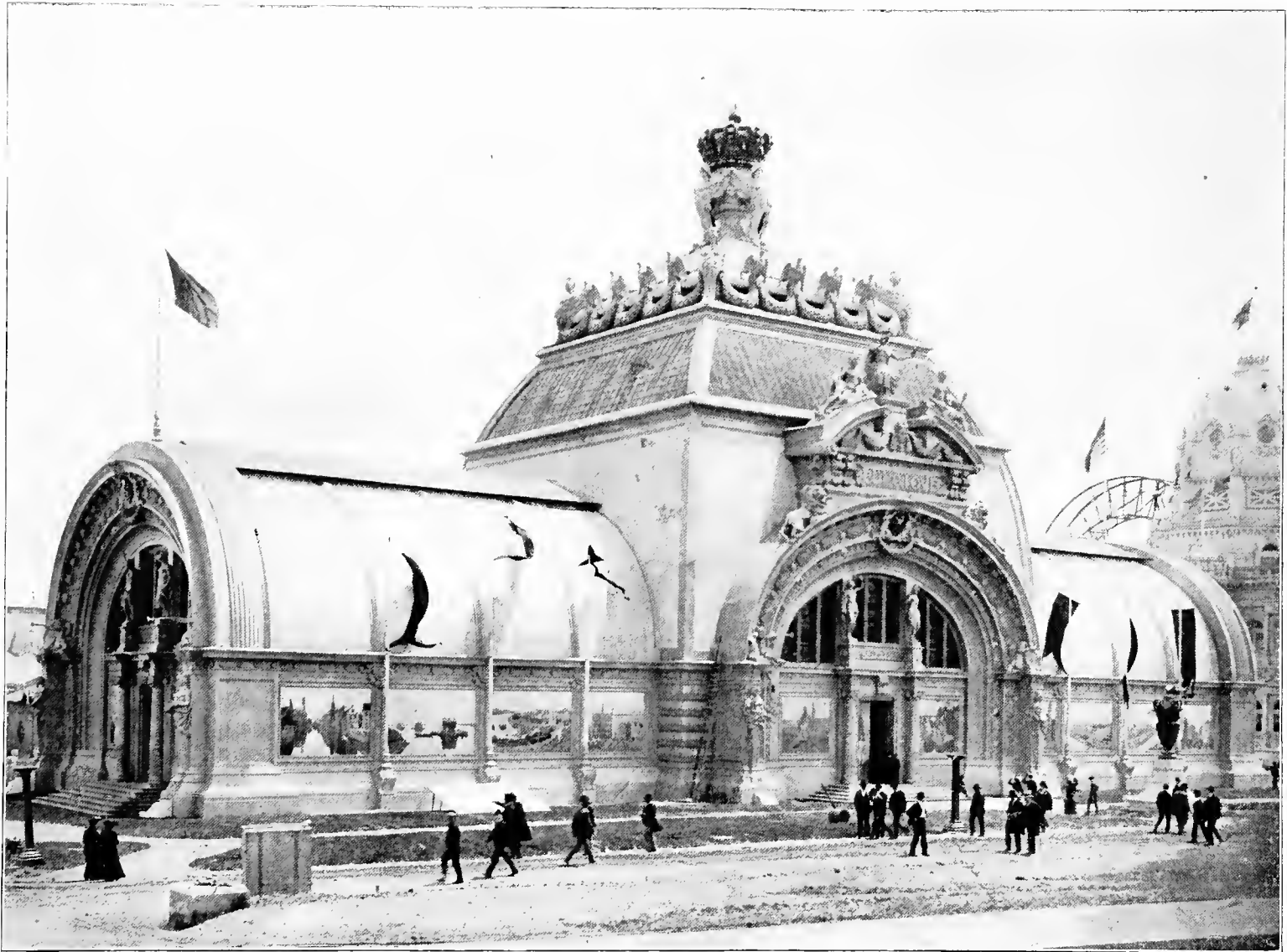
THE BELGIAN BUILDING.
